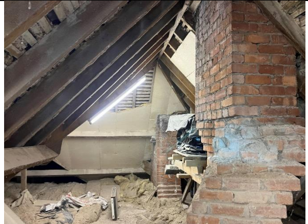
Photograph 2: internal loft space with lighting
