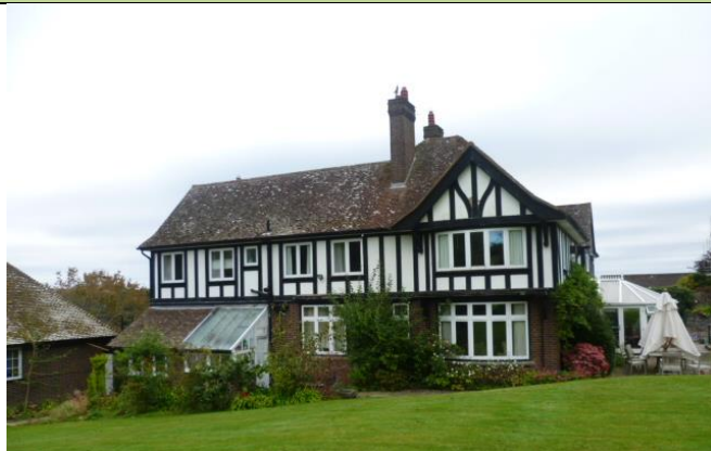
Photograph 5: Existing dwelling (B1, centre) with garage (B2, left)
