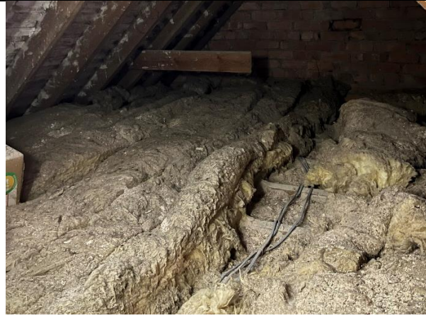
Photograph 4: loft insulation is present throughout
