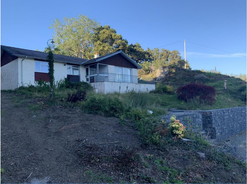
A. Bungalow at Crud-yr-Awel (surveyed for bats).(2020)
