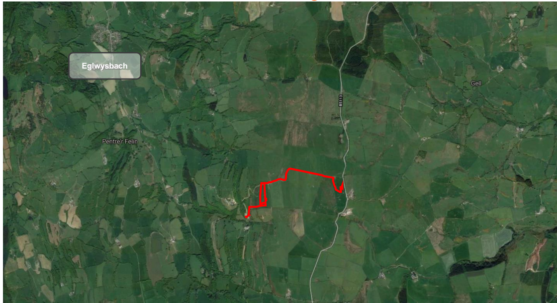
Figure 2.1. An aerial image of the site in relation to Eglwysbach and its wider surroundings.
