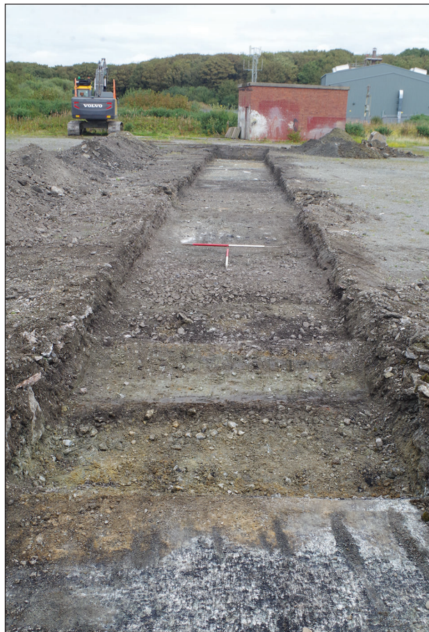
Figure 8: Trench 2 (prior to sondage excavation), tarmac 203 in foreground, view from south-west, 2 x 1 m scales
