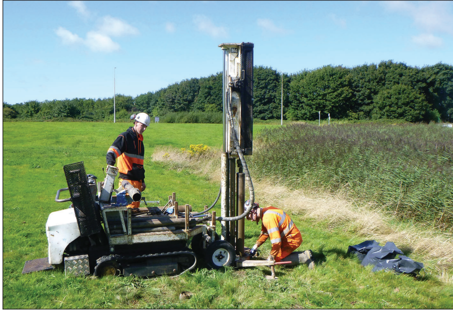
Figure 3: Excavation of borehole WA-01, view from south-east
