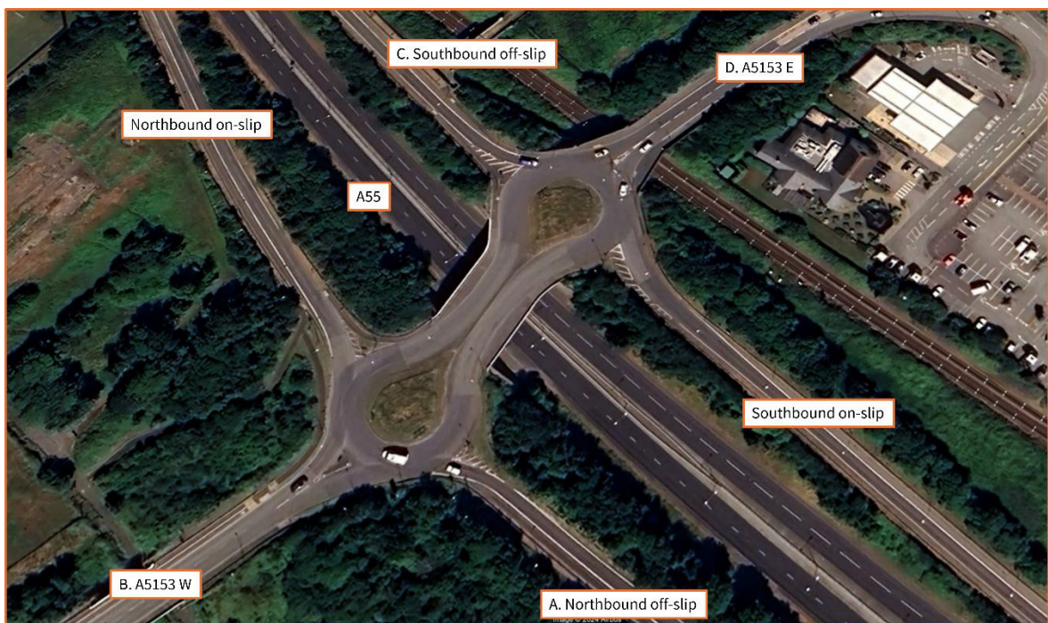
Figure 16: A55 Junction 2 Ty Mawr Interchange
