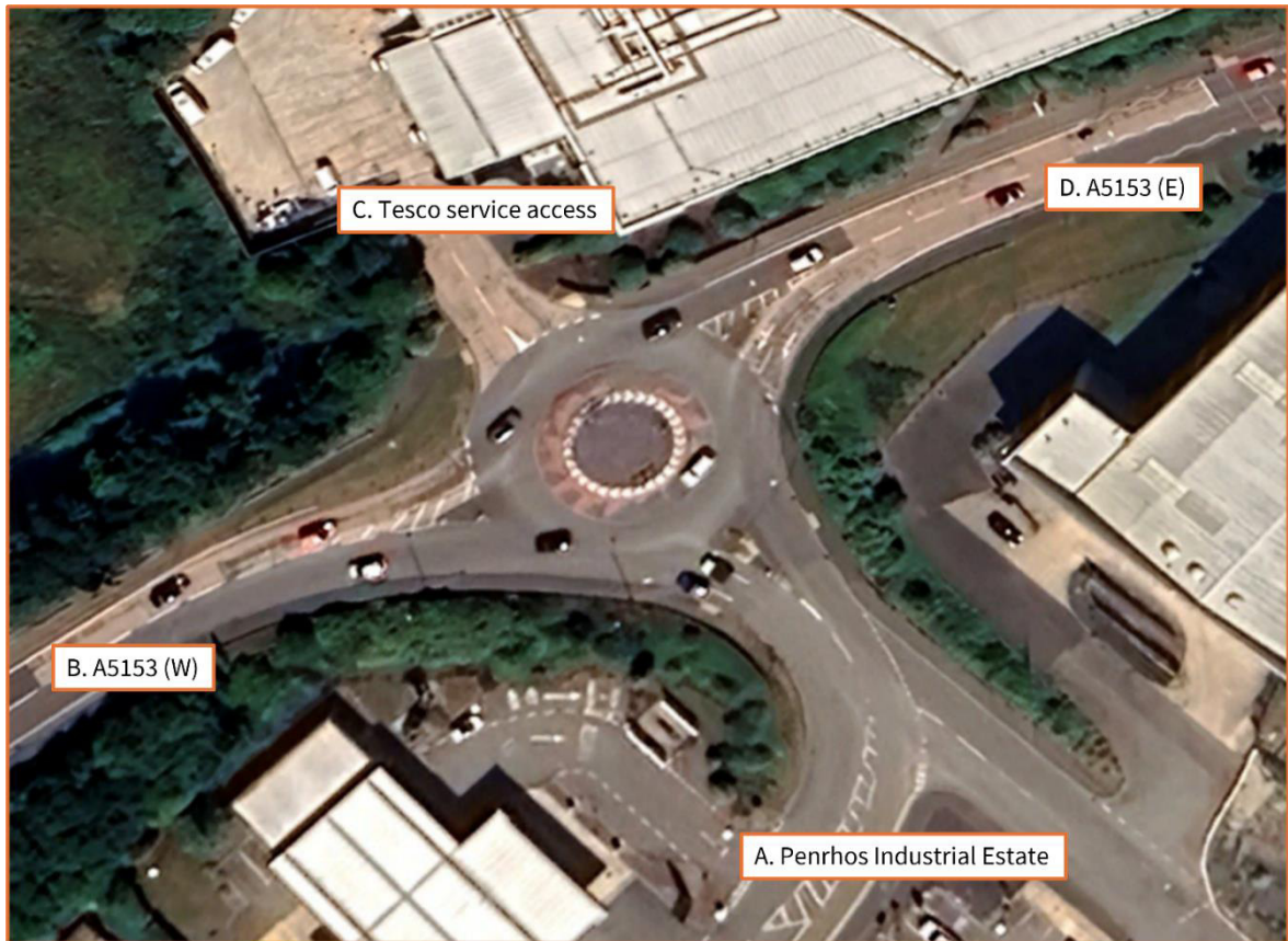
Figure 18: A5153/Penrhos Industrial Estate western roundabout
